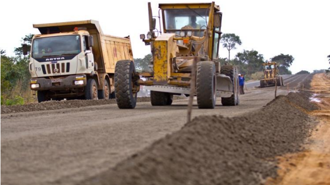
FIGURE 13: CRUSHED STONE BASE CONSTRUCTION
