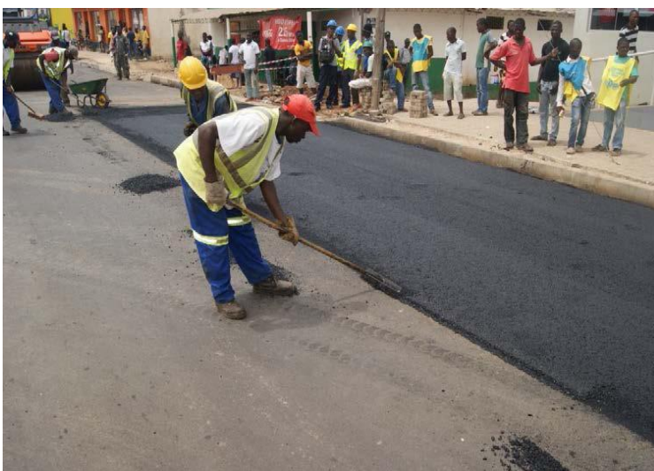
FIGURE 16: PLACEMENT OF ASPHALT CONCRETE
