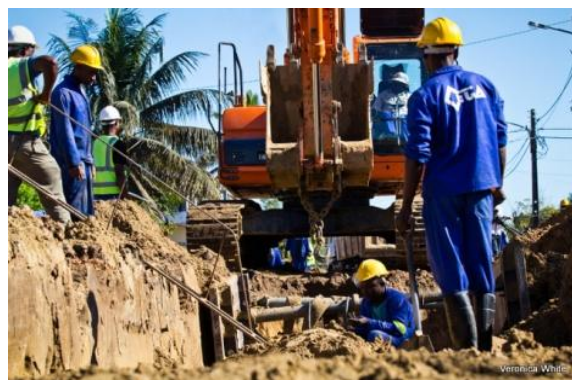
FIGURE 6: CONSTRUCTION OF STORM WATER CHANNEL
