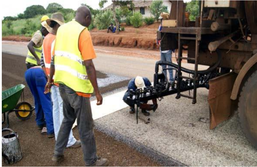
FIGURE 15: PLACEMENT OF SECOND SEAL
