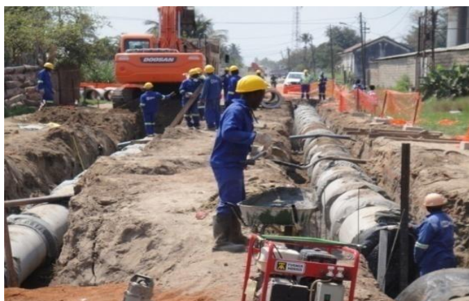
FIGURE 10: CONSTRUCTION OF STORM WATER PIPE SYSTEM
