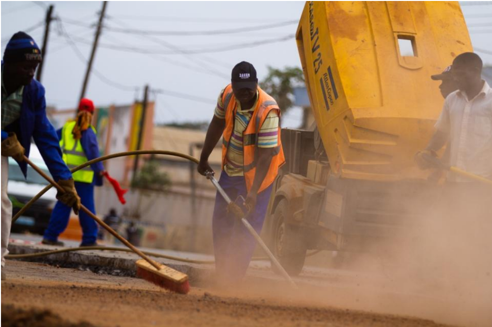
FIGURE 18: CLEANING OF ROAD PLATFORM
