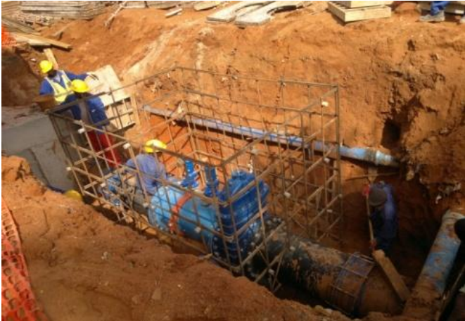
FIGURE 4: CONSTRUCTION OF VALVE CHAMBER
