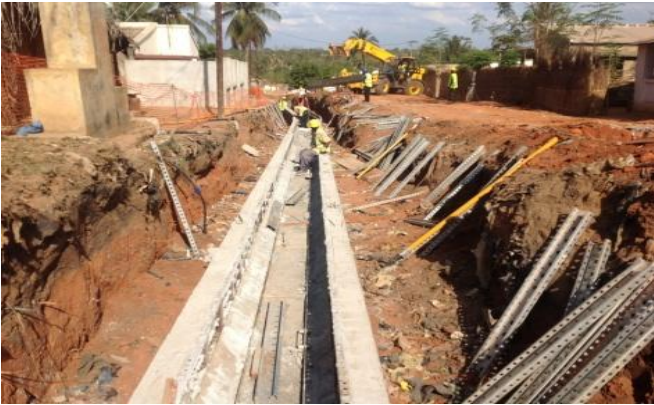
FIGURE 8: CONSTRUCTION OF DRAINAGE CHANNEL
