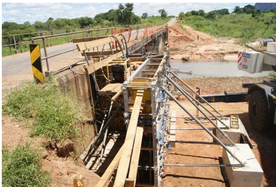
FIGURE 14: PREPARATION WORKS FOR BRIDGE WIDENING
